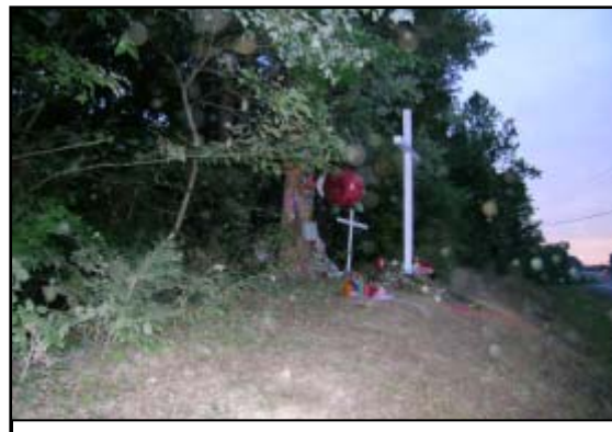
Figure 5. Tree impact at the top of the embankment.
