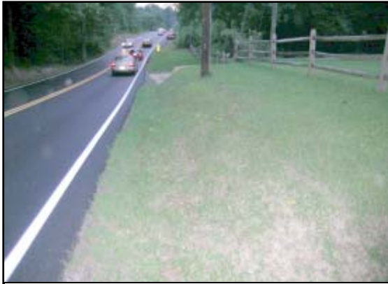
Figure 2. Right side road departure.
