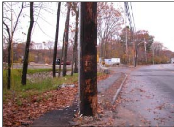
Figure 4. Struck 43 cm (17.0") diameter utility pole.
