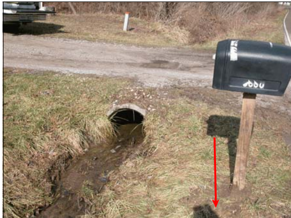
Figure 3: Overview of impacted culvert and mailbox, arrow shows location of old mailbox post
