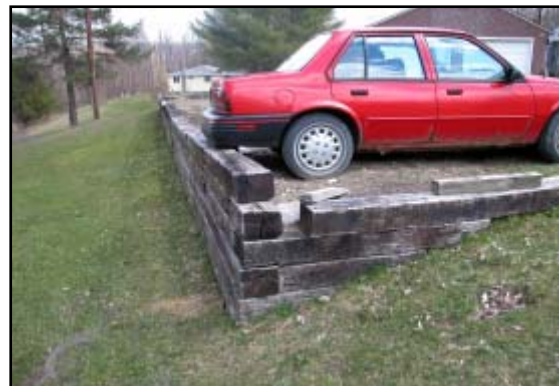
Figure 4. Area of impact with the wood retainer wall,
