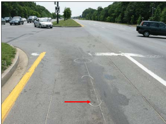
Figure 6: Point of impact in southwestbound left turn lane, arrow shows gouge marks in pavement from crash
