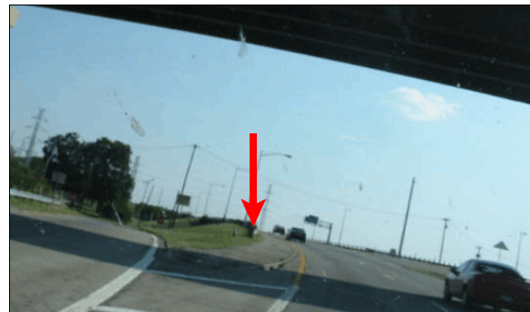
Figure 3: Approach of case vehicle southwest bound into gore, arrow shows impacted guardrail (repaired)
