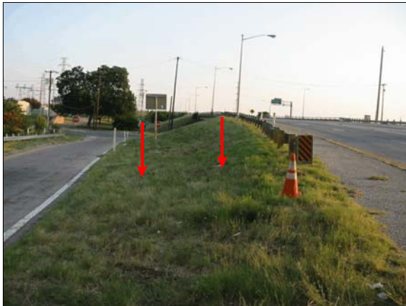
Figure 6: Overview of impacted guardrail (repaired), arrows show locations of exit ramp sign post bases
