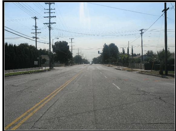
Figure 4. Approach to area of impact (south)
