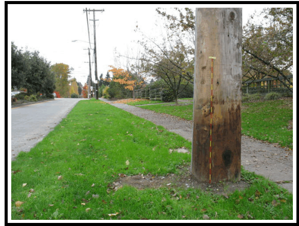
Figure 7. Impacted pole (east)
