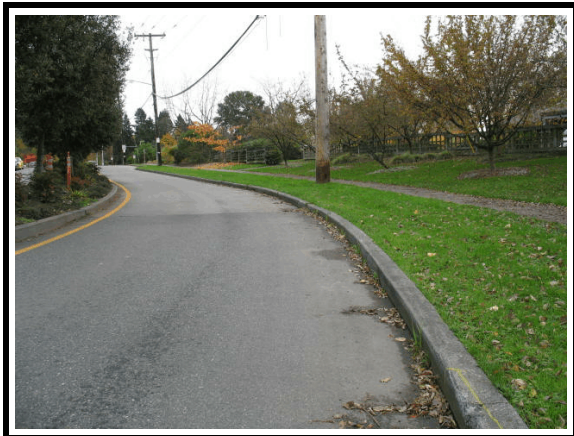
Figure 5. Approximate roadway departure area (southeast)
