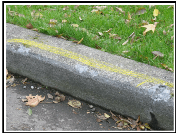
Figure 6. One section of curb damage
