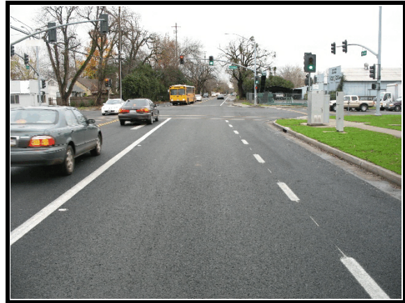
Figure 3. Approach to area of impact (southeast)
