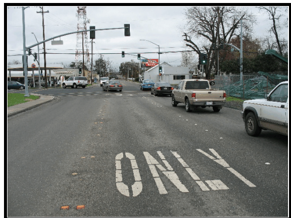
Figure 2. Approach to area of impact (northeast)
