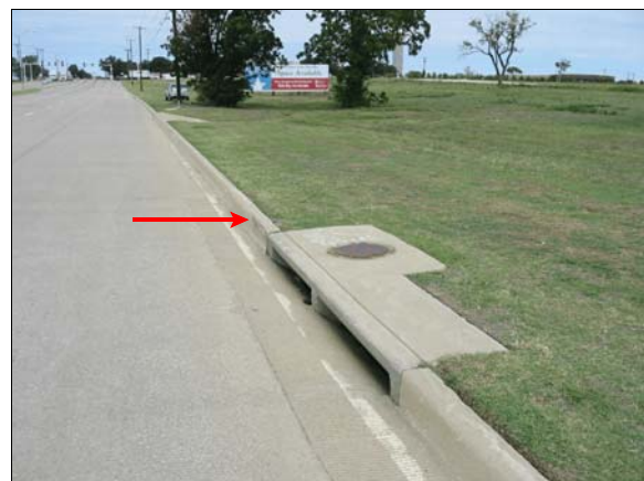
Figure 2: Approach of case vehicle to curb impacts, arrow shows location of right front wheel curb impact
