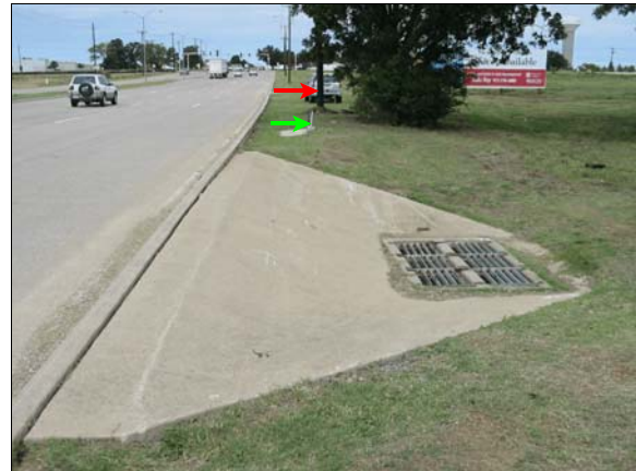
Figure 3: Approach of case vehicle across drainage basin to telephone utility box impact (green arrow) and utility pole impact (red arrow)
