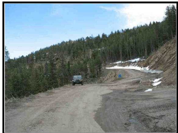
Figure 2. Eastbound approach to area of roadway departure
