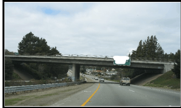
Figure 3. Area of road departure and impact with center guardrail (north)
