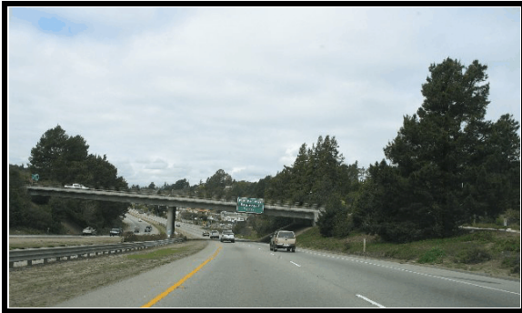
Figure 2. Approach to area of road departure (north)
