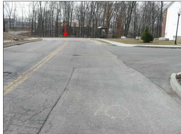
Figure 1: Approach of Lincoln southbound to road departure (arrow), number on pavement indicates meters to fire hydrant impact
