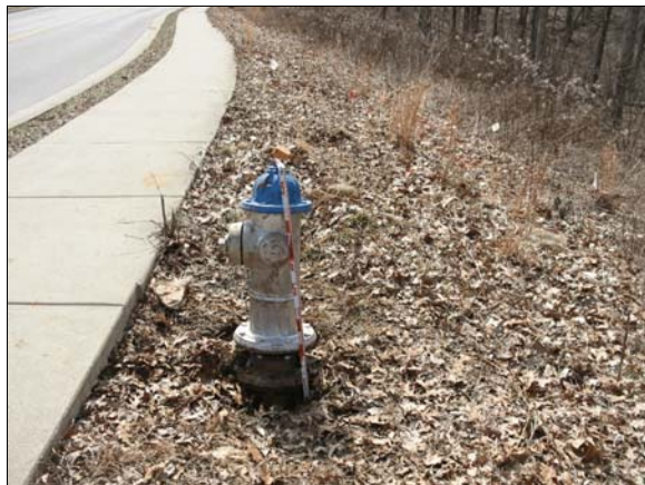
Figure 4: Location of impacted fire hydrant (repaired)
