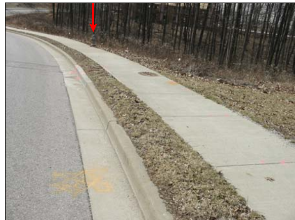
Figure 2: Area of Lincoln roadway departure, arrow shows impacted fire hydrant (repaired)
