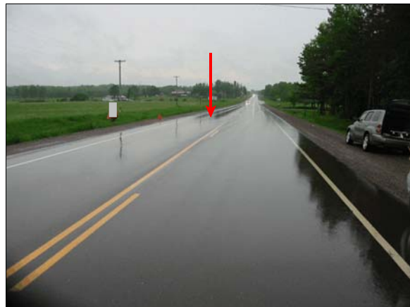
Figure 1: Approach of Jeep northbound to impact area (arrow)
