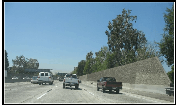
Figure 3. Approach to area of impact
