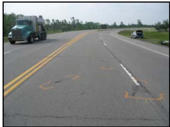
Figure 6: Left front and left rear gouge marks.
