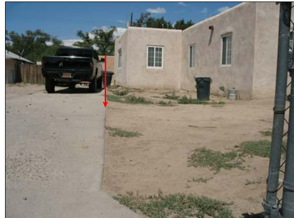
Figure 2: Arrow shows rise from yard to driveway edge
