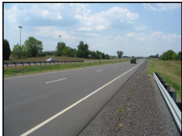
Figure 2: Southward view of the crash site.
