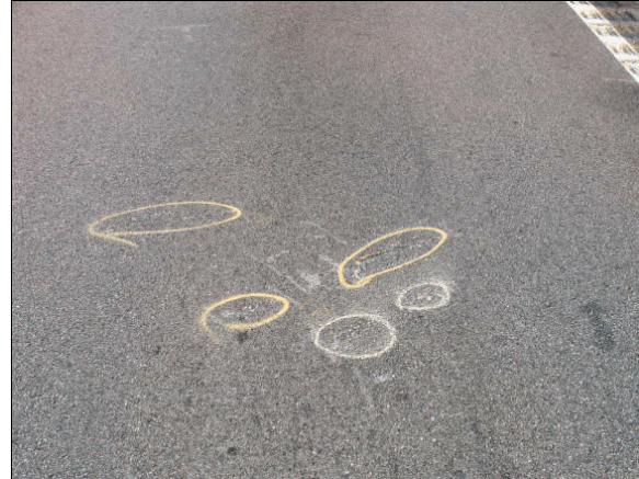
Figure 6: Impact gouges in eastbound lane
