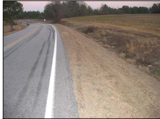
Figure 3 - Area of roadside departure.
