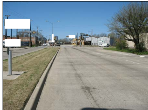
Figure 3: Approach of Mitsubishi to the intersection
