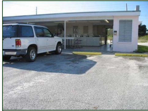
Figure 2. Look back view of the incident site.
