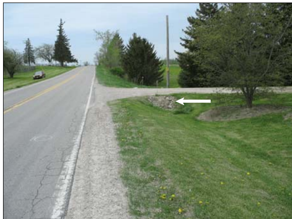
Figure 3: Arrow shows location of initial impact with culvert and area of rollover initiation
