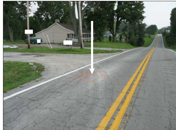
Figure 4: Arrow shows impact gouges in northbound lane
