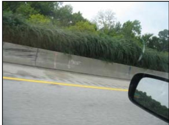
**Figure 3: Depicts the contact evidence to concrete barrier wall from the Ford's first event**
