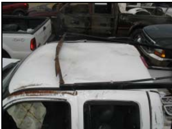
Figure 5: Rollover damage to the roof.
