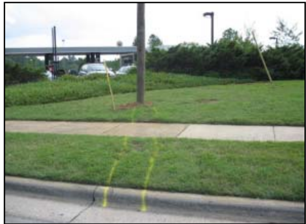
Figure 5. Curb and utility pole impact.
