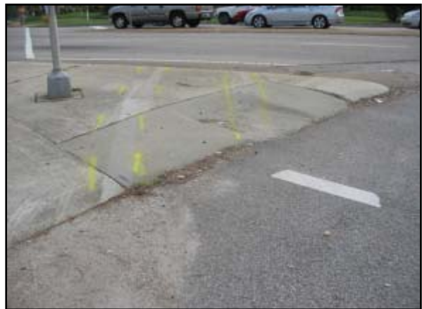
Figure 3. Saturn's travel across the concrete gore.
