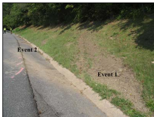
Figure 4: View depicting the errant trajectory of the Ford and the gouges that resulted from Events 1 and 2.
