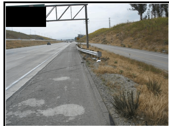
Figure 3. Area of rollover, guardrail contact, and pole impact (skid on shoulder not related to this crash)
