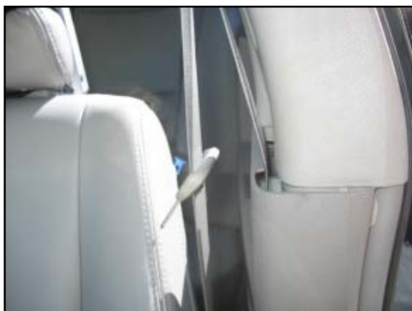
Figure 10. Dislodged left B-pillar trim panel.
