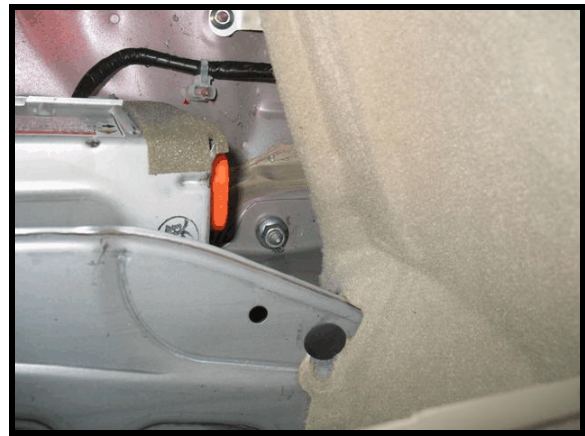
Figure 9. Traction battery service plug
