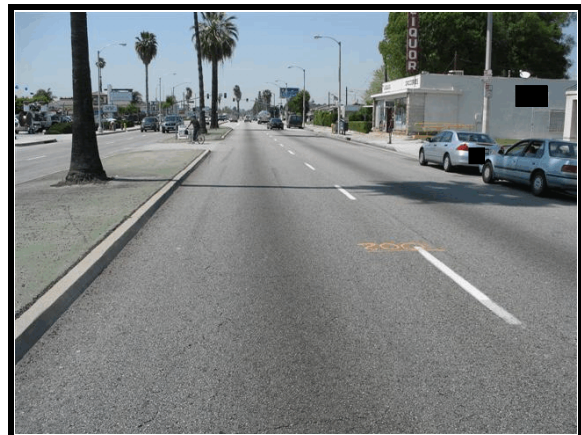
Figure 2. Westbound approach to area of impact
