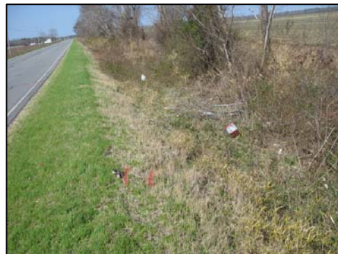
Figure 3: Embankment and rollover site
