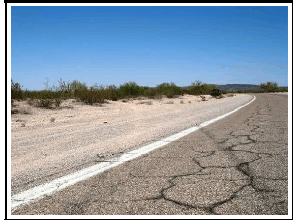
Figure 7. View showing travel path from roadway departure to trip point
