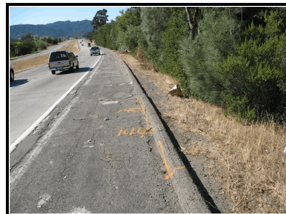
Figure 3. Area of roadway departure and impacts with asphalt curb
