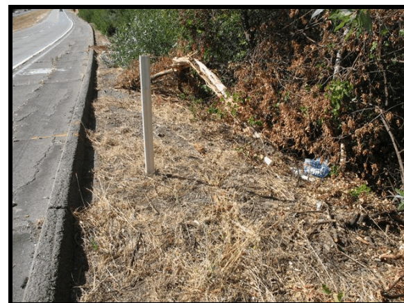
Figure 4. Area of impact to delineator and tree
