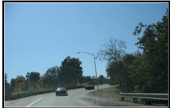
Figure 2. Transition roadway (ramp)
