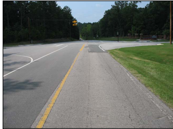
Figure 2: Southbound approach to the intersection.
