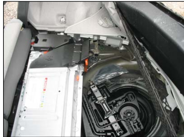
Figure 8: Left lateral view of the right floor deformation aft of the hybrid battery.
