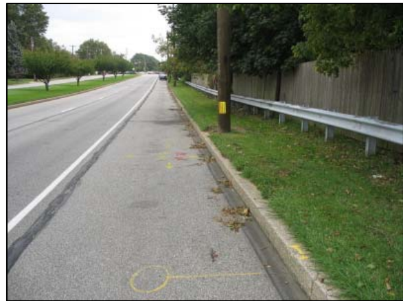
Figure 3: Trajectory view of the curb strike and utility pole impact.
