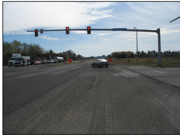
Figure 3: Area of initial impact depicting post-crash roadway resurfacing
