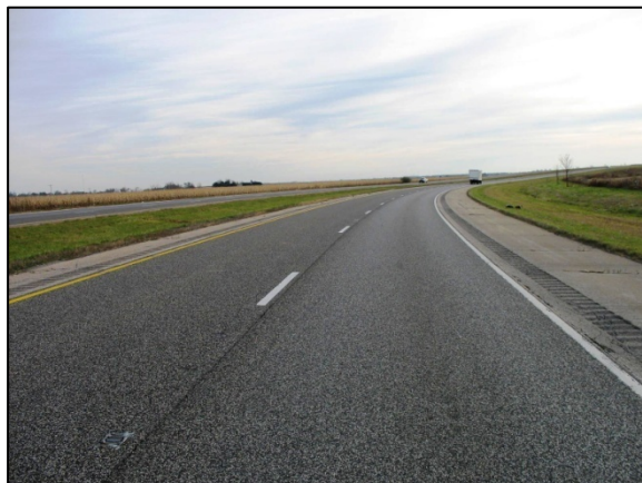
Figure 2: Southbound view of the roadway depicting the pre-crash travel path of the Scion.
