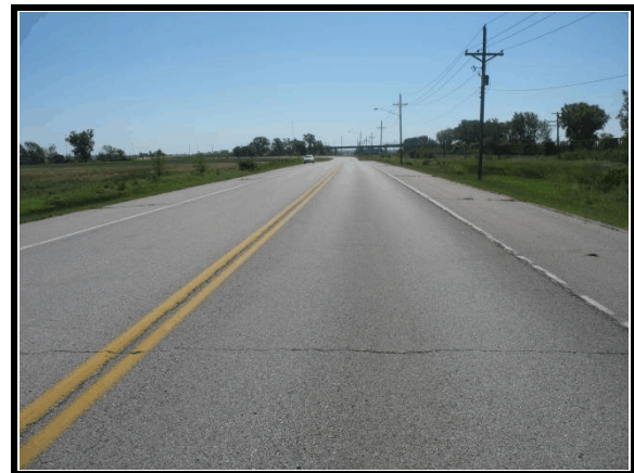
Figure 2. Eastbound travel lane
