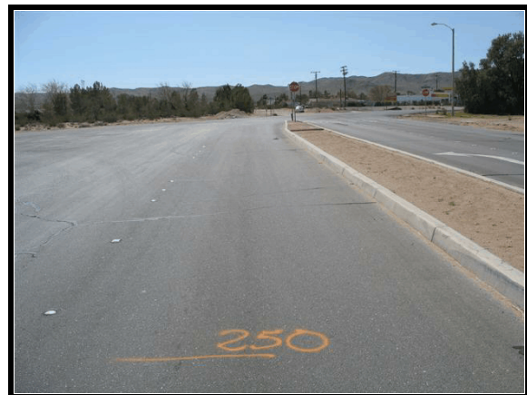
Figure 2. Southbound approach, 76.2 m (250 ft) from point of impact
