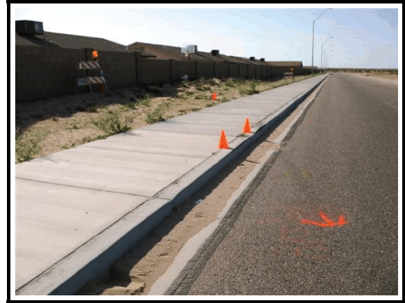
Figure 3. Area of impact showing tire skid mark in foreground, curb impact in mid-ground, and pole impact in background
