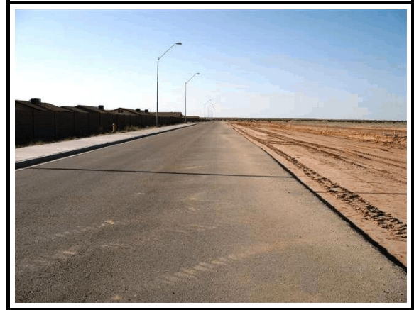
Figure 2. Crash site, southbound approach
