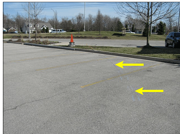
Figure 6: Approach to impacts with curb and concrete light pole; arrows show right front tire mark
