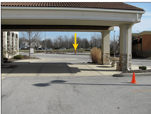
Figure 5: Lexus traveled under covered customer drop off area of restaurant; arrow shows location of impacted concrete light pole
