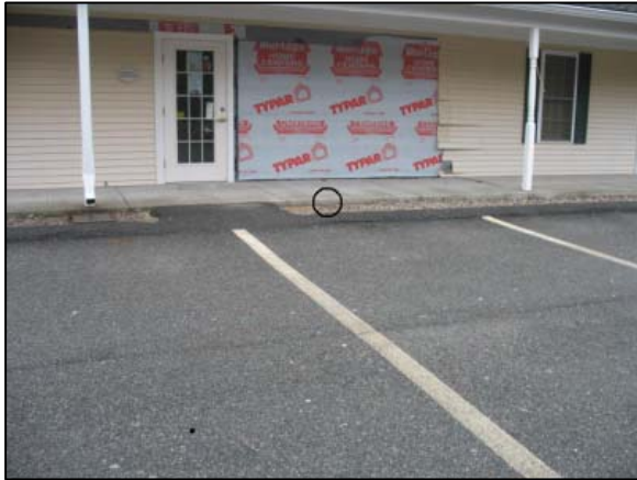
Figure 2: Trajectory view of the Toyota approaching the building and the general area of impact.
