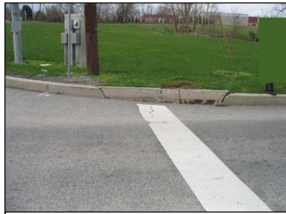
Figure 4: View of the fractured and displaced northeast curb.
