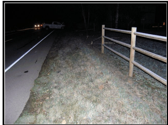
Figure 3. Area of impact with fence (Event 1)
