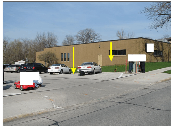
Figure 3: Approach through parking lot entrance to parking space (arrow on left); arrow on right shows location of impact on the building
