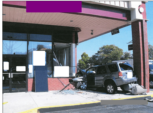
Figure 11: View northeast to final rest position of the Ford and the damage to the building from the impact
