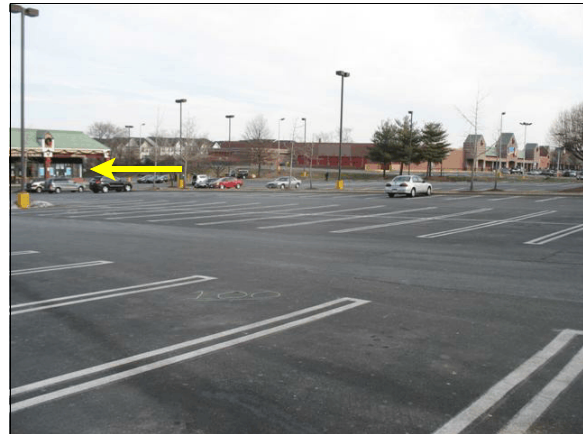
Figure 3: Approach through the parking lot to the impact with the building; arrow shows the impacted building (view northeast)
