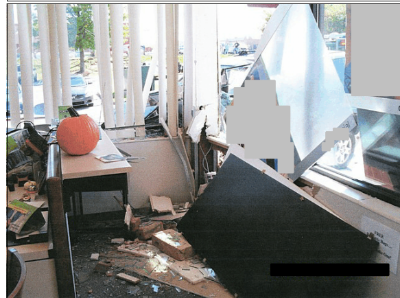
Figure 12: On-scene photo of the interior damage to the building from the impact by the Ford; view to southeast
