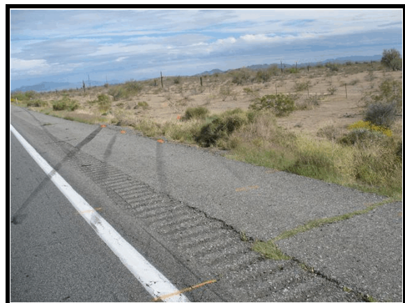
Figure 5. Right side roadway departure
